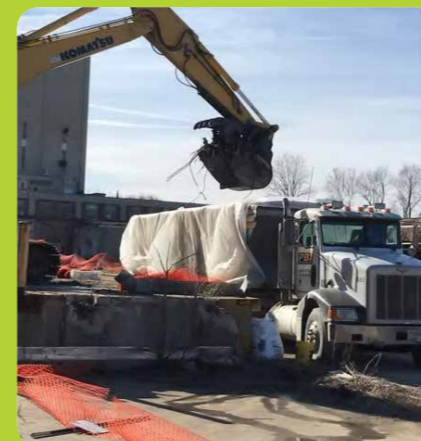
Material loaded into lined plant for safe controlled transport to landfill.
