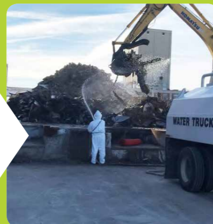
Water spray mist is used for dust mitigation.
